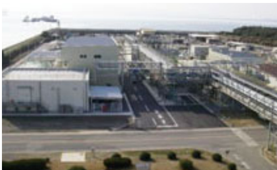
Activated sludge treatment facility using the oxygen aeration method
