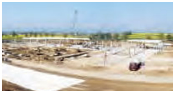
Construction site of the new company in Poland
