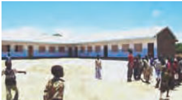
School building constructed in Tanzania
