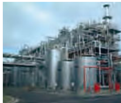
Caprolactam plant at the Ehime Works
