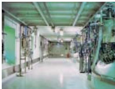
Pharmaceutical manufacturing facilities
